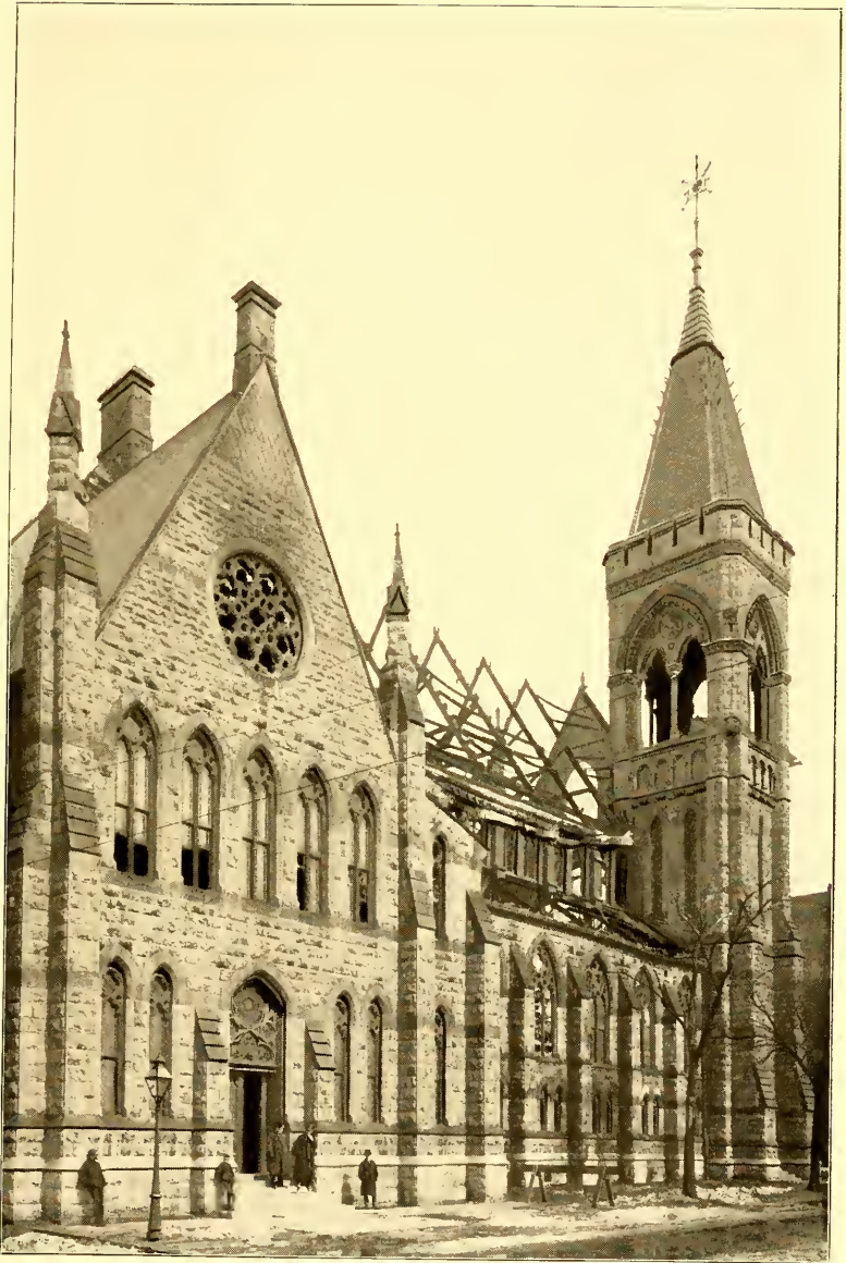
THE SECOND PRESBYTERIAN CHURCH, N. W. CORNER OF MICHIGAN AVENUE AND TWENTIETH STREET. DESTROYED BY FIRE THURSDAY NIGHT, MARCH 8, 1900. THIS PICTURE WAS TAKEN THE DAY FOLLOWING THE FIRE.
